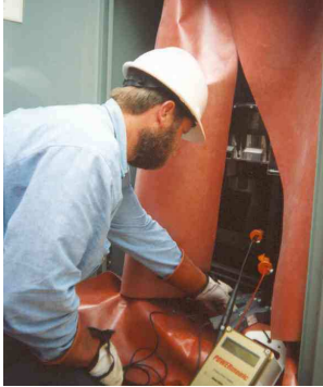
Fig 15 – Use of insulating mats in switchboard application
